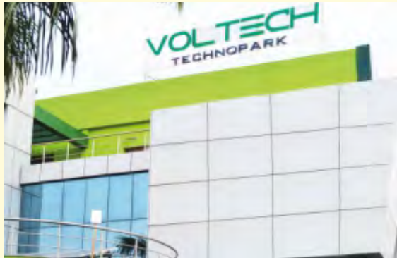
Techno Park 1 Switchgear, Solar & Battery Charger
