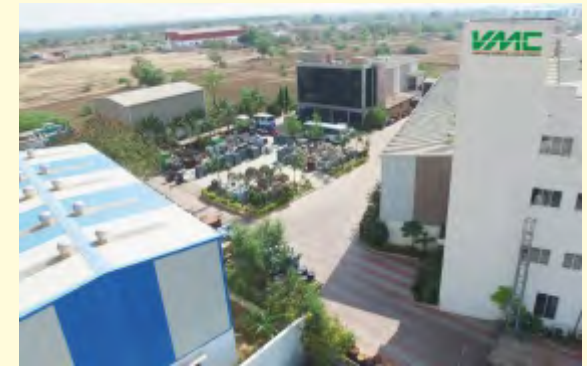
Techno Park 3 Distribution & Power Transformer
